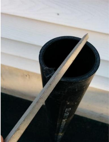
3. Continuing filing until the file reaches it's full depth (top side of the file even with the top of the pipe).
